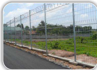
Pagar Wire Mesh Wire Mesh Fence
